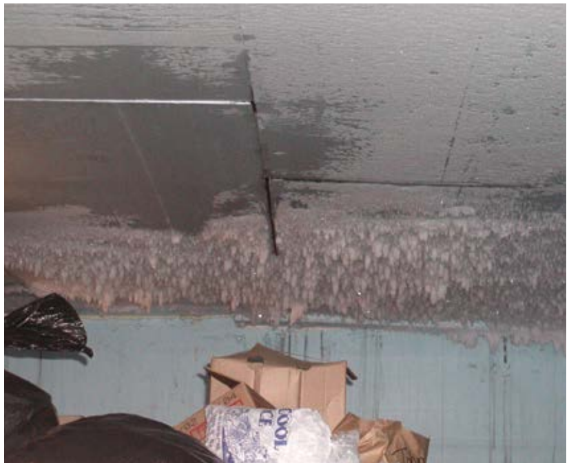
Condensate on the ceiling of a cooler can drip onto contents below, creating a food safety risk.
