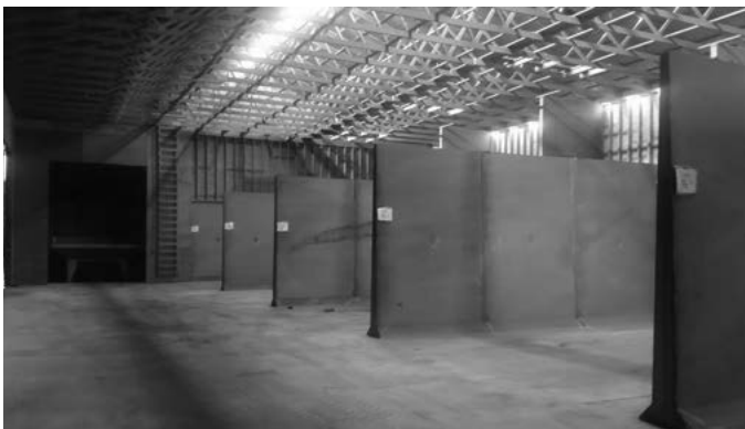
On-farm dry bulk fertilizer storage bins
