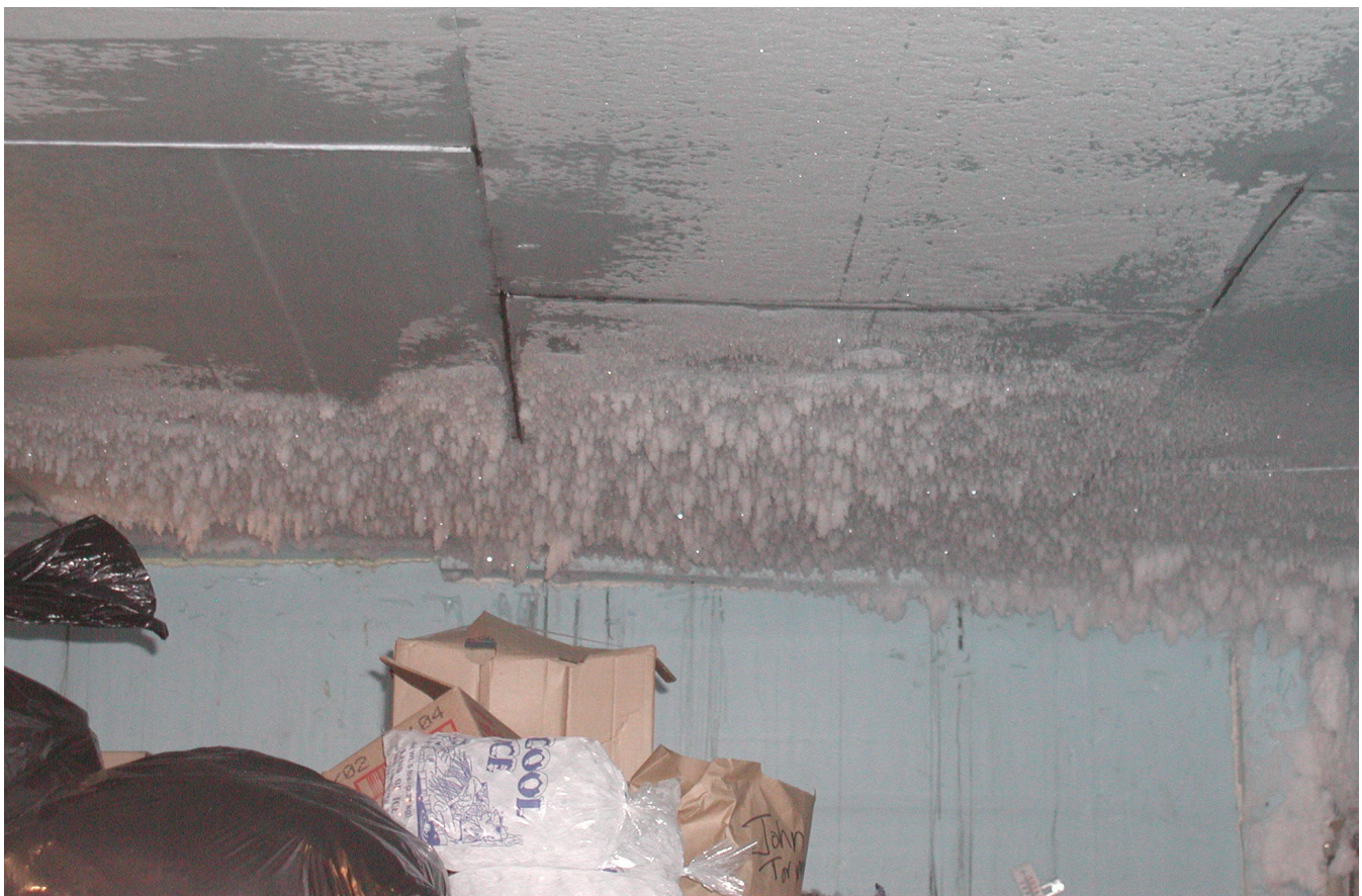
Condensate on the ceiling of a cooler can drip onto contents below, creating a food safety risk.
