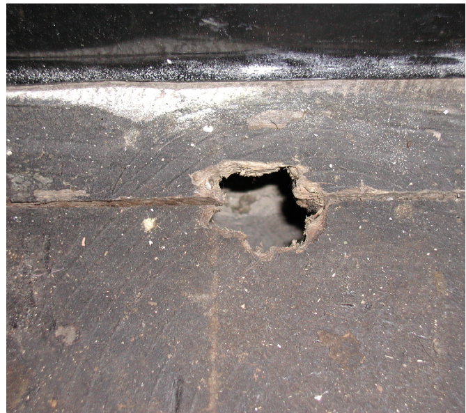
In the left photo, the door does not close tightly, leaving a gap between the door and the floor that is unacceptable in a meat processing facility as it could permit the entry of vermin; In the right photo, a hole in the ceiling needs to be repaired.
