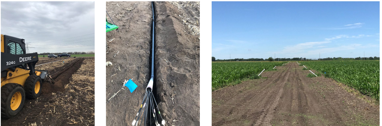
Figure 2. Suction cup lysimeter installation at the Rosholt Farm in 2020.
