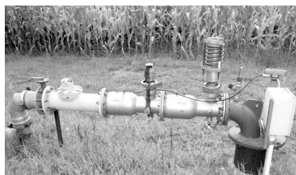
Center Pivot irrigation system equipped with two back-check valves for the application of fertilizers and/or pesticides when connected to a non-potable water supply.
