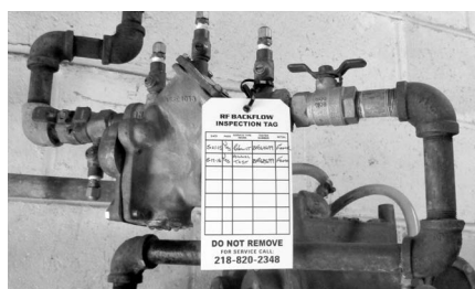
Greenhouse irrigation system equipped with a Reduced Pressure Principle device (RPP or RPZ) for chemigation when connected to a potable water supply.
