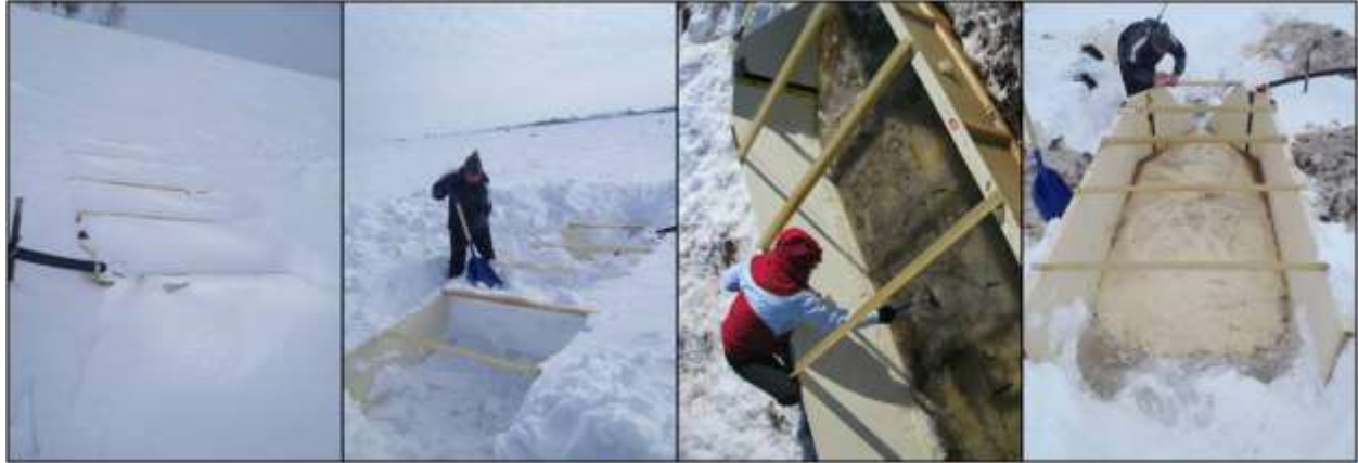
Figure 14. Progression of flume cleaning. 1) Shovel and remove excess snow. 2) Carefully melt and chip out any ice. 3) Clear upstream and downstream flow paths.
