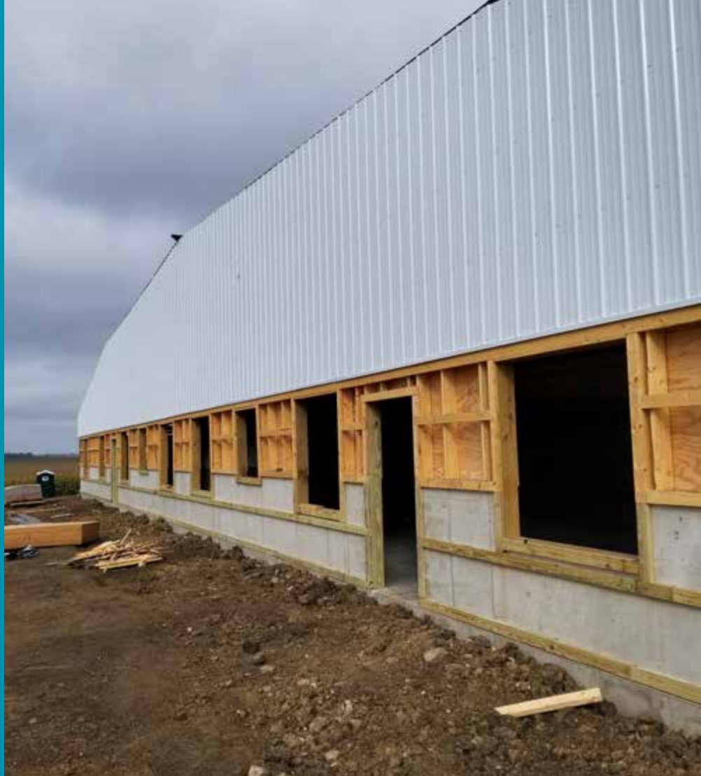
Barn construction during summer, 2017.
