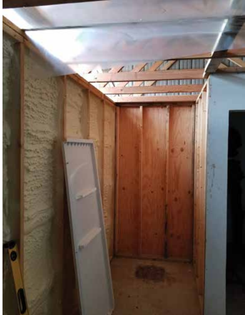
Open walls during construction show spray foam insulation after installation.
