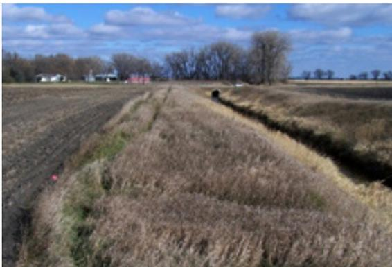
Figure 1. Example of a buffered drainage ditch.
