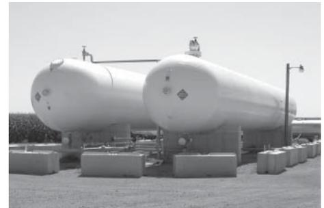
Anchored/stabilized concrete barriers with access gaps of no more than 3 feet. Warning markers to a height of 3 feet are required for barriers that are less than 3 feet in height.
