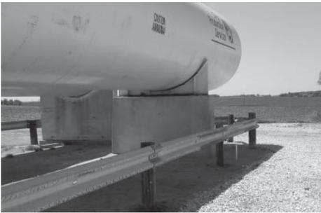
DOT approved guardrail attached to posts at a height of at least 3 feet. Each post is positioned every 10 feet and is anchored into the ground by a 12 X 48 inch concrete foundation.
