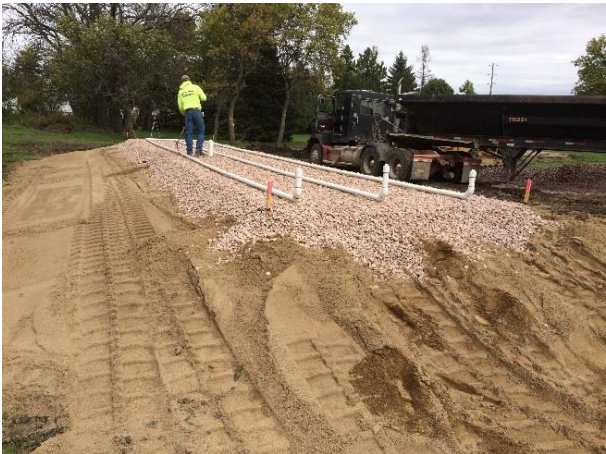
Figure 22. Installation of a typical septic tank and mound drain field, Watonwan County.
