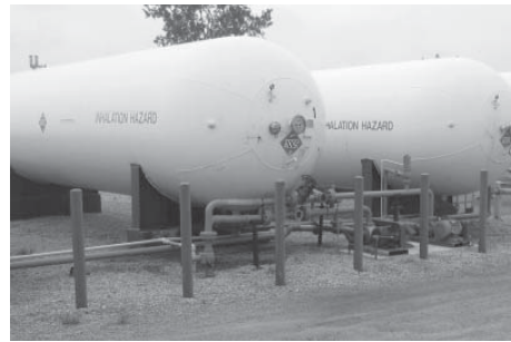
Steel posts at least 3 feet high, positioned every 4 feet. Each post is anchored into the ground by a 12 X 48 inch concrete foundation.
