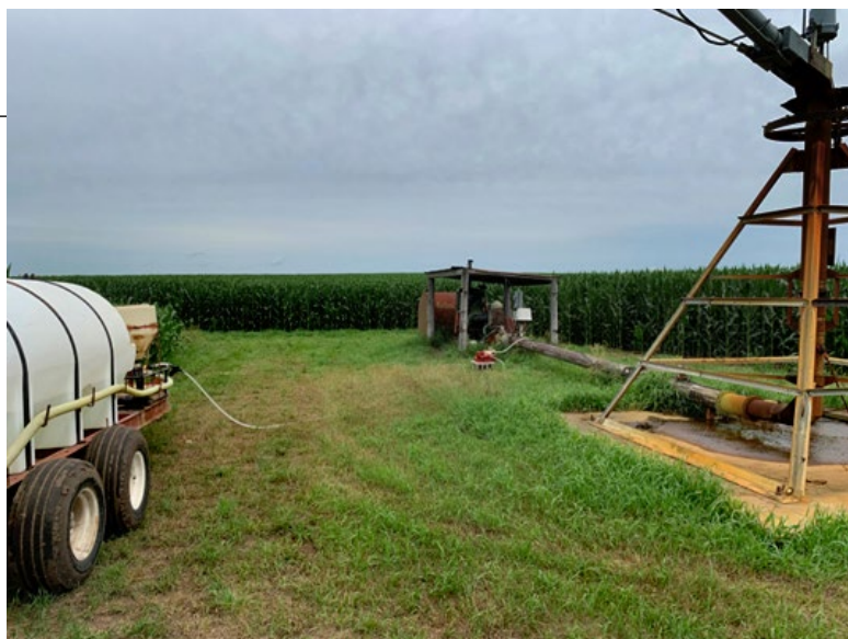
Chemigation supply well and fertilizer supply tank greater than 20 feet from well
